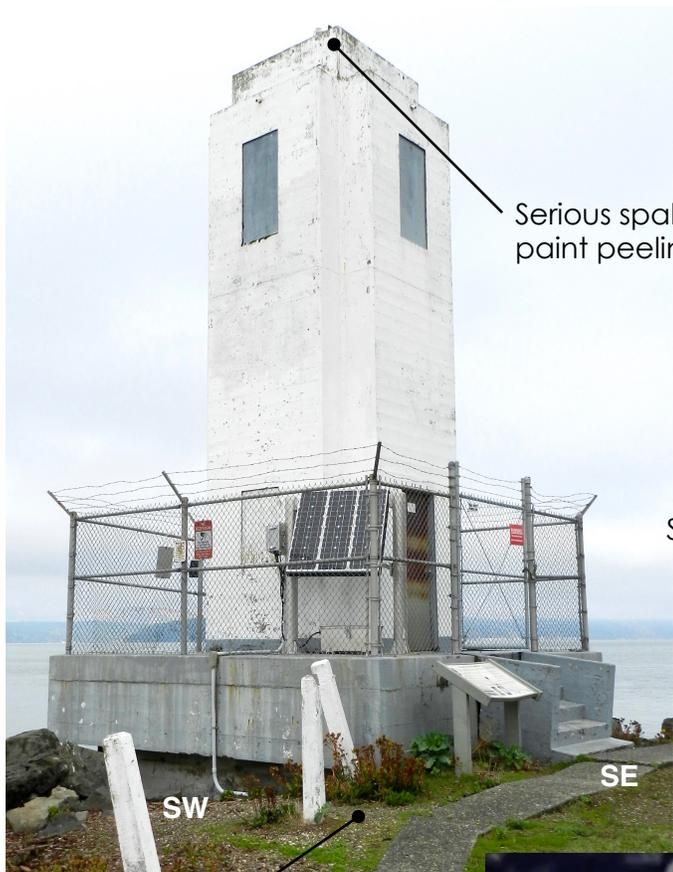
Serious spalling; paint peeling
