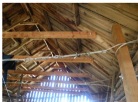
Plates temporarily held in place with steel cables with turnbuckles
